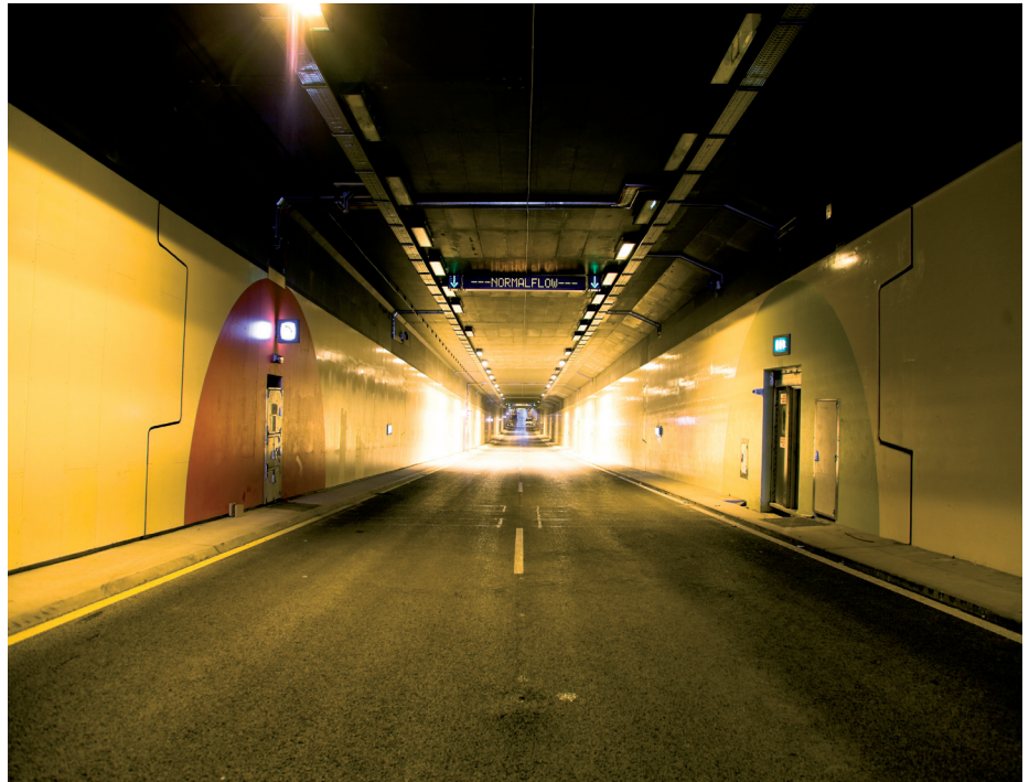
A view inside the Limerick Tunnel
