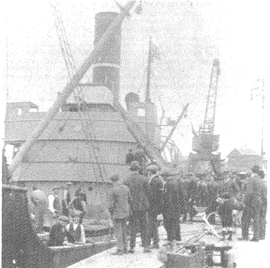
Timber for the Shannon Scheme being unloaded at the Limerick Docks on September 1925.
